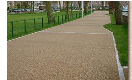
PAVING TYPE F: Resin Bound footway has longer life span and is porous. Resin bonded footway as used in Dolphin Yard
