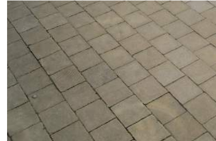
PAVING TYPE B: Yorkstone setts 100 (w) x 150-250mm (l) - Sawn cut - Marshalls Cromwell option for footways and parking bays within lightly trafficked areas when used with Yorkstone slabs
