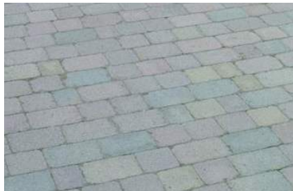
PAVING TYPE D: Concrete setts Marshalls Tegula 80mm thick x 160mm width, 3 size lengths for carriageway paving. (Parliament Sq)
