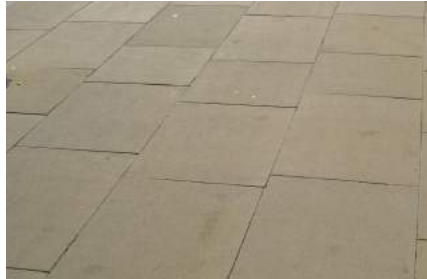
PAVING TYPE A: Yorkstone paving slabs - 300, 450, 600mm widths x 50mm x random lengths. If vehicle overrun is likely use 75mm thick slabs random lengths. Flame textured
